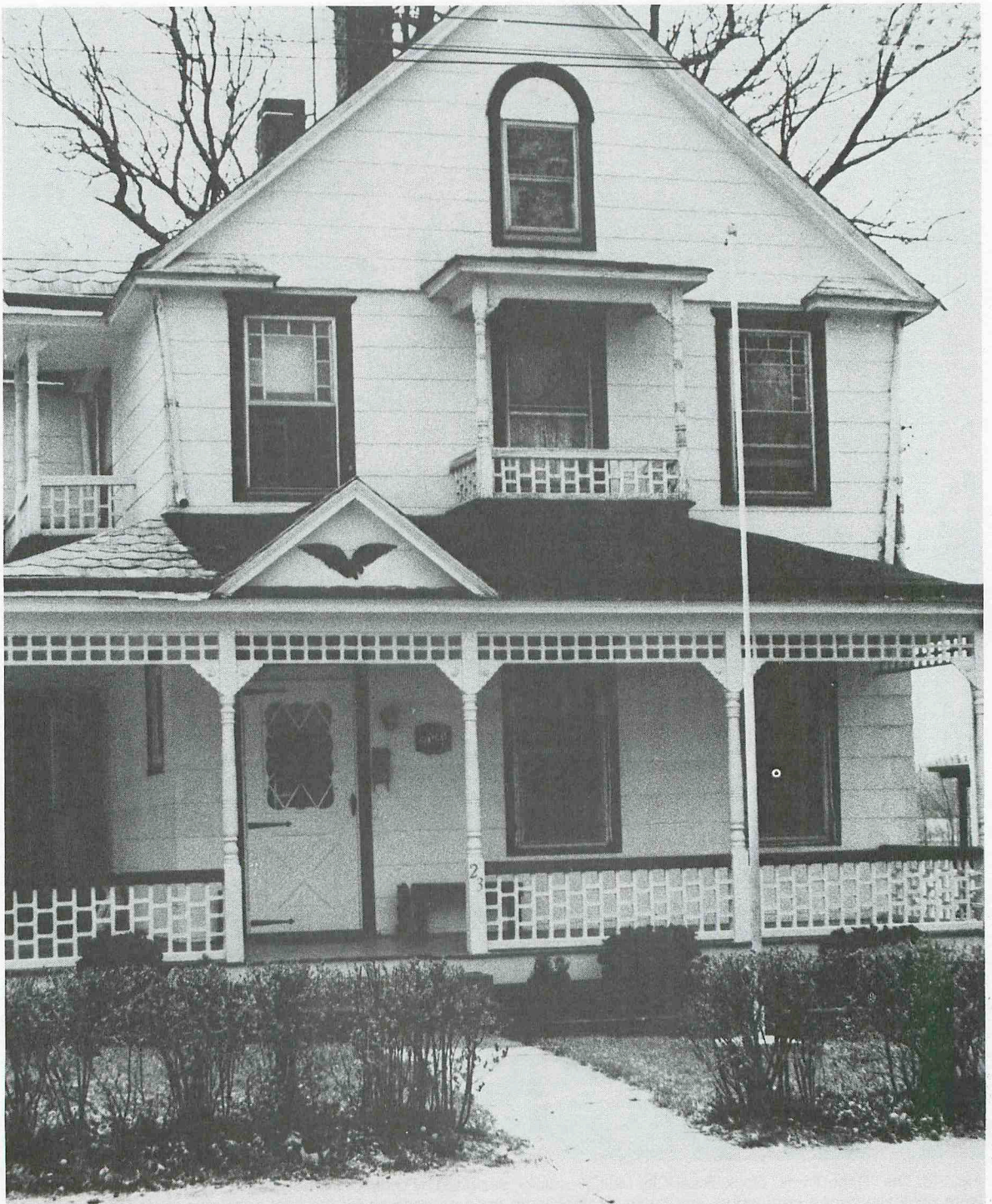
Fig. 7-2. The pillars are combined with lattice work and extend even to the sides of the house in the old tradition.
