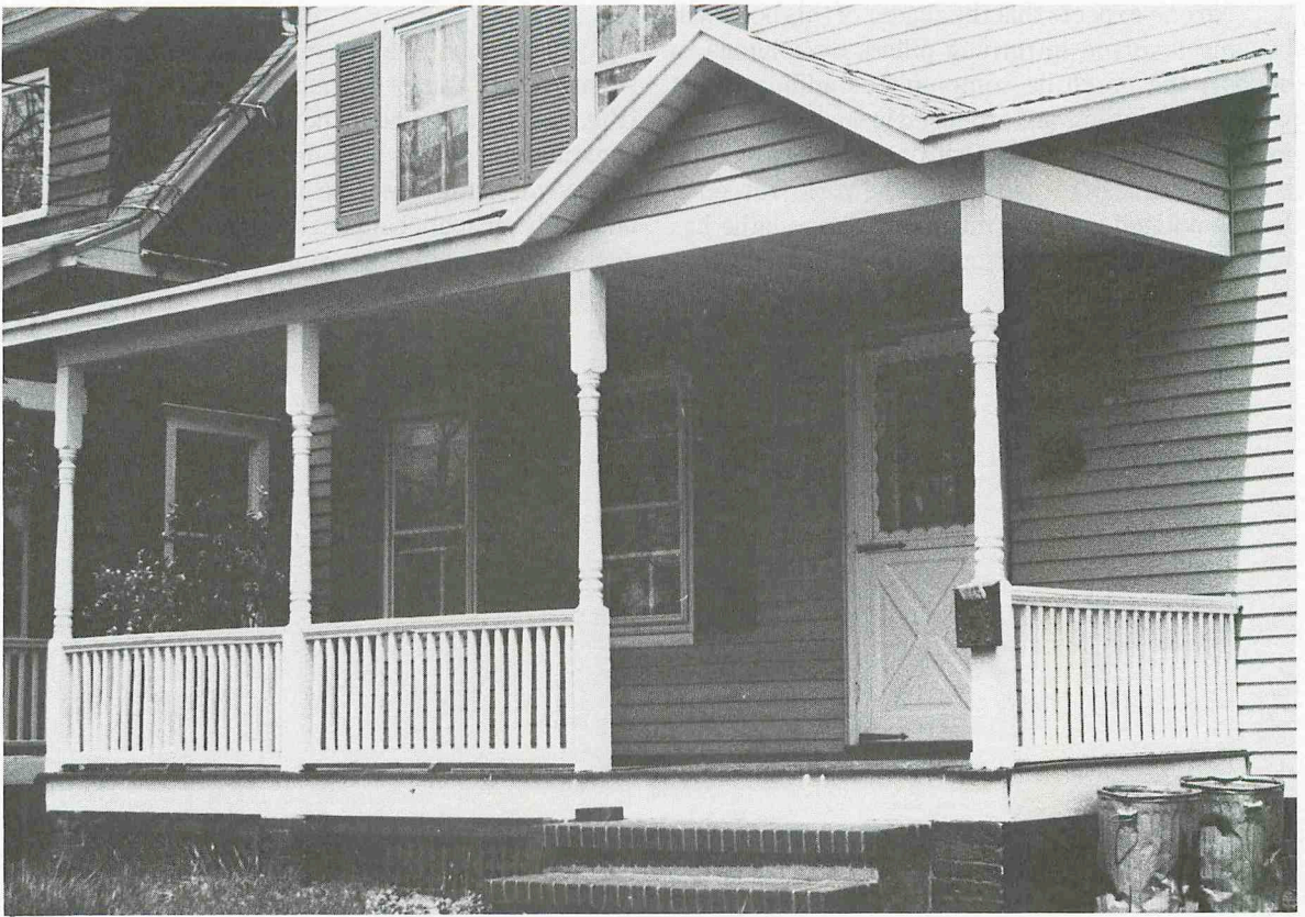
Fig. 7-4. These columns are prevalent throughout New Jersey, indicating that they may be mass produced for small builders.
