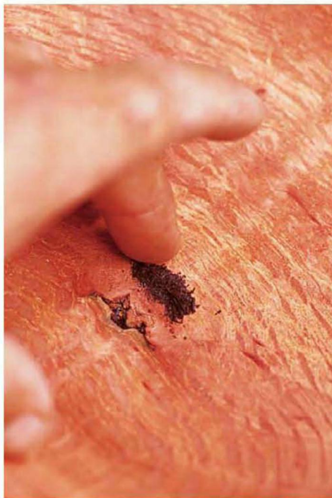
Fill very small gaps and defects with fine dust before adding a few drops of thin cyanoacrylate adhesive (Super Glue) to set it in place.
