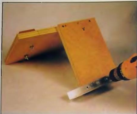
27. Attach the aluminum rail to the upright plywood.
