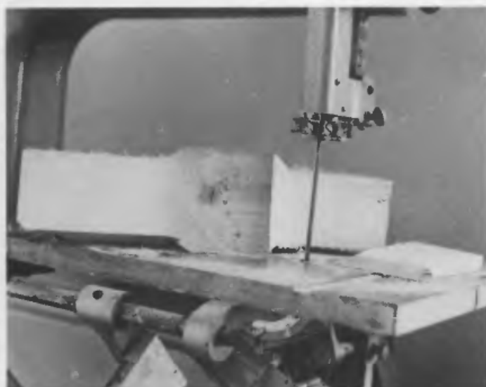
Fig. 10 Using a 15in. [381mm.] bandsaw to prepare a blank for turning a leg which has a maximum turned diameter larger than the pummels
