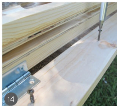
14 Drive no. 6 woodscrews, centered under each row of holes, to act as stops as the discs are dropped.
