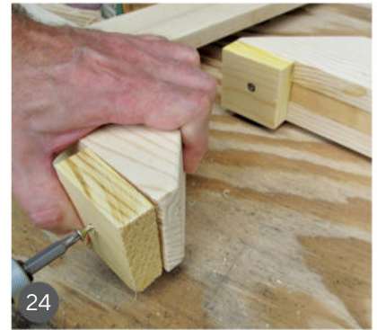
24 Attach the foot pads to the leg assemblies.
