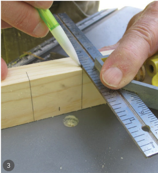
3 Mark the location for the wide notch or housing.
