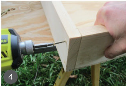
4 Screw the sides to the ends.
