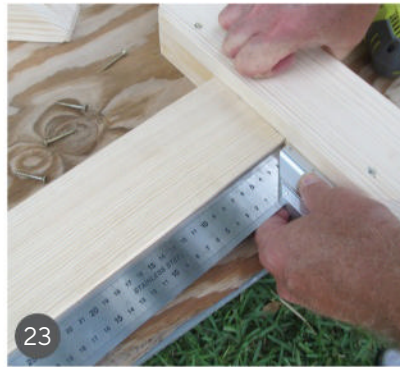
23 Insert the uprights into the feet, making sure they're square before fastening them with screws.
