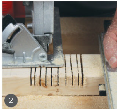
2 Using a straightedge and a circular saw set to half the thickness of the wood, make multiple cuts between the lines. (Note the pencil lines either side of the joint to locate the saw fence.)
