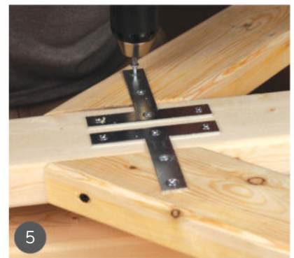
5 Screw on the T-brackets.
