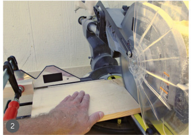
2 Cut 28 tiles, making sure the end of each tile is tight against the stop block before making the cut.
