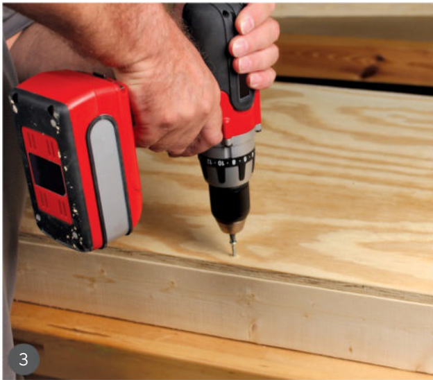
3 Screw the top board onto the frame.
