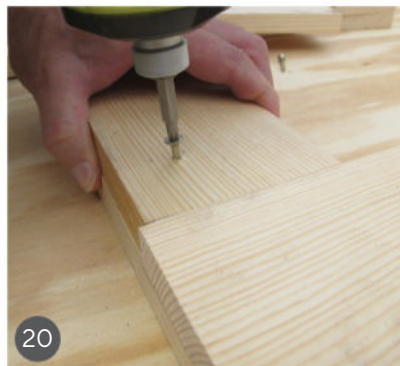
20 Attach the filler pieces, using the upright as a guide for placement.
