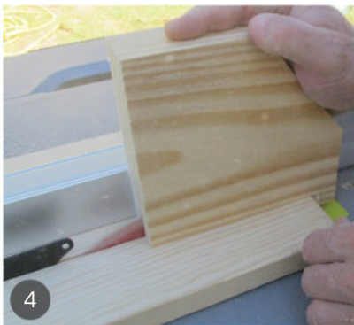
4 Rip the frame pieces to width at the tablesaw, using a push block for safety.
