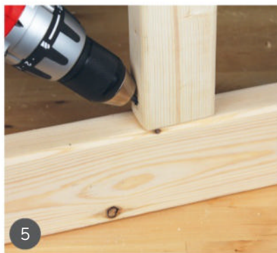
5 Drill diagonal holes for screwing the uprights to the feet.
