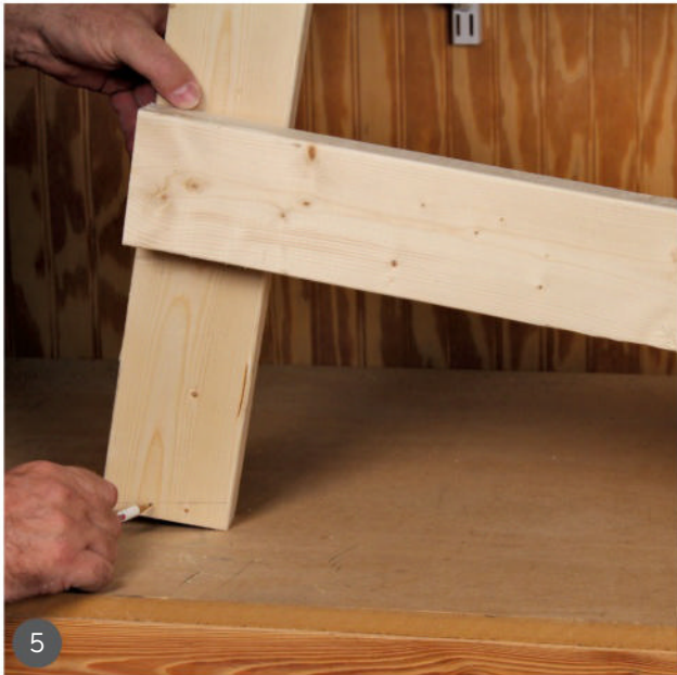
5 Mark the angles on the legs, then cut them.
