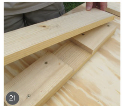
21 Attach the outer face with glue and screws.
