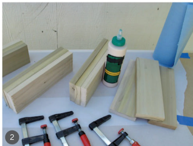
2 Get everything ready for gluing up the three layers to form each mallet head.
