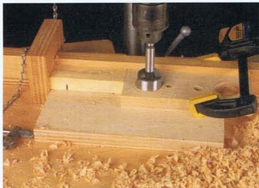
Photo D • Drill 1\frac{1}{8} -in.-diameter holes in the blanks to create the interior wheel-well curves on the stacked fender blanks.
