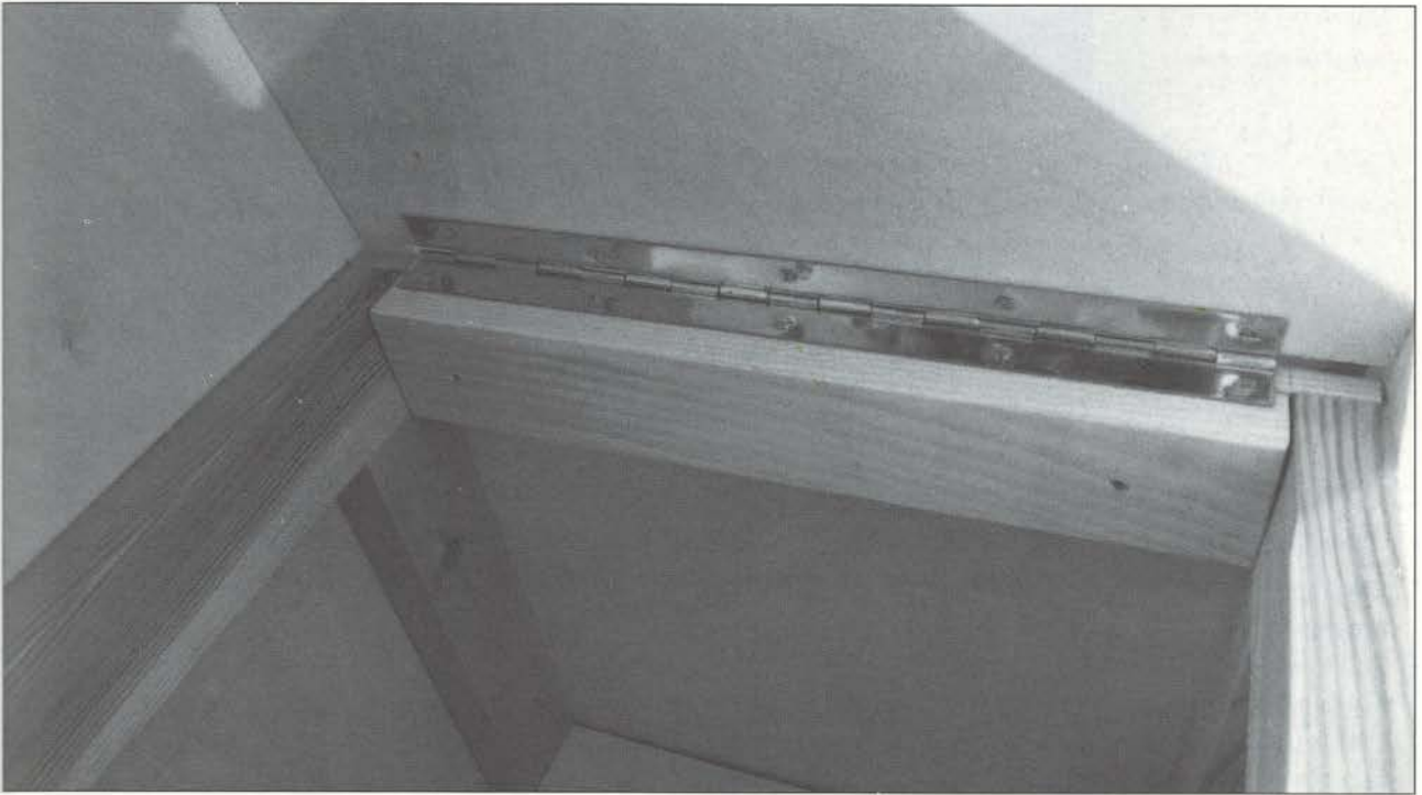
Fig 13.8 The seat board and hinge-support batten are screwed into the piano hinge.
