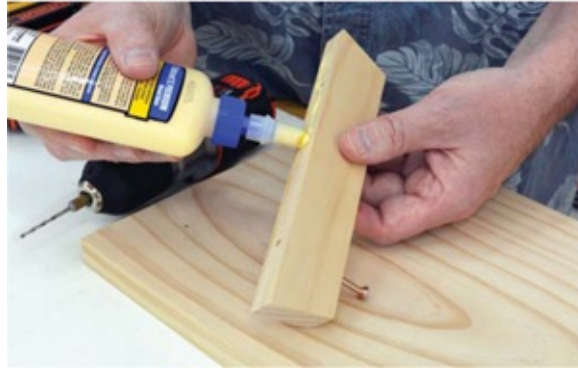
Photo 9 Glue and screw the support foot about 1" from the bookrack's open end.
