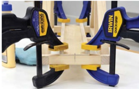
Photo 13 Glue the trough sides into place, then glue and clamp the trough assembly to the bottom of the frame.
