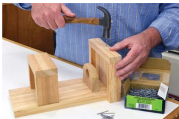
Photo 10 Frame the feeder shelf with 1- \frac{1}{2} " cedar glued and nailed into place.
