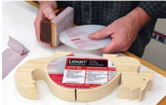
Photo 6 Sand off any burrs or sharp edges with a sanding block.
