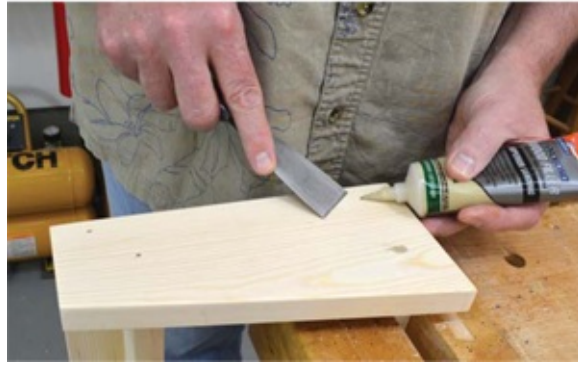
Photo 6 Touch up the nail holes and any other blemishes with wood filler.
