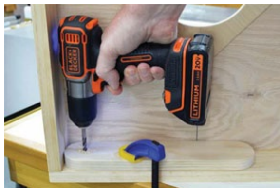
Photo 13 Drill the pivot holes for the legs with them clamped into place inside the top corners of the game board.
