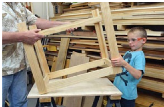
Photo 7 Center the up-ended leg set on the underside of the benchtop.
