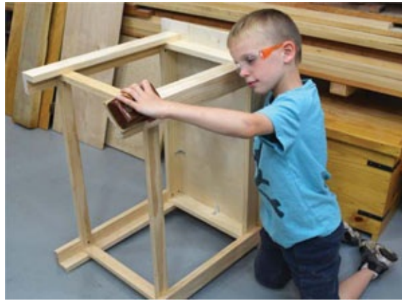
Photo 9 A final once-over with a sanding block will smooth any sharp edges.
