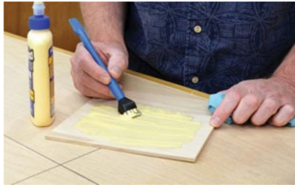
Photo 2 Spread glue on the back of the plywood hole reinforcement.
