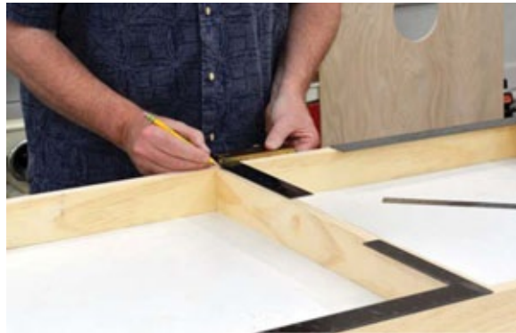
Photo 7 Lay out the location for the middle frame piece at 24" on each side of the frame assembly, and check for square.
