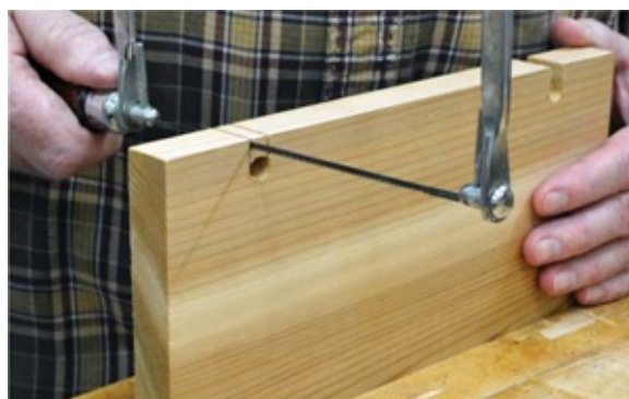
Photo 5 A coping saw makes quick work of the two roof notches.
