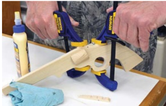
Photo 7 Glue and clamp the clothespin into place and allow to dry thoroughly.
