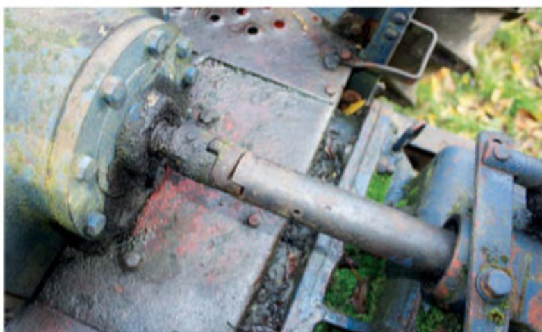
The drive shaft, minus the safety cover, showing the shear pin location (protecting the pump from overload).
