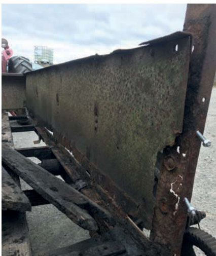
Corrosion, as you might expect, was extensive.
