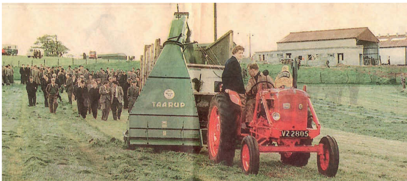
This picture shows a green Taarup S 1500 being demonstrated at Loughry College in 1958. It is powered by a Nuffield Universal Four. Photo: Courtesy of Billy Armstrong.
