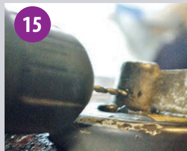
Drilling out the old broken roll pin with a tungsten drill bit.
