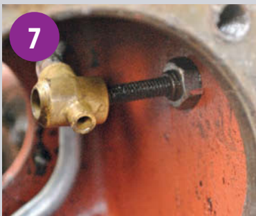
Here is the bolt I should have released before removing the valve block.
