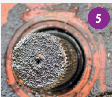
With the steel collar behind the arm removed, there is the seal.
