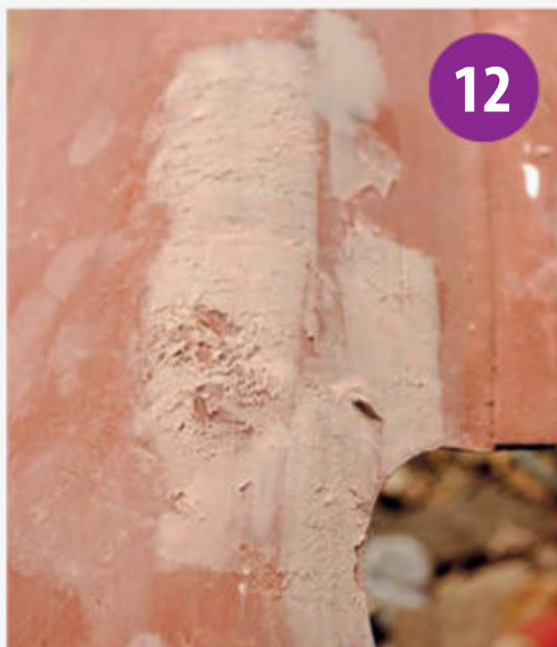
Apply the filler, leaving it proud of the surface.
