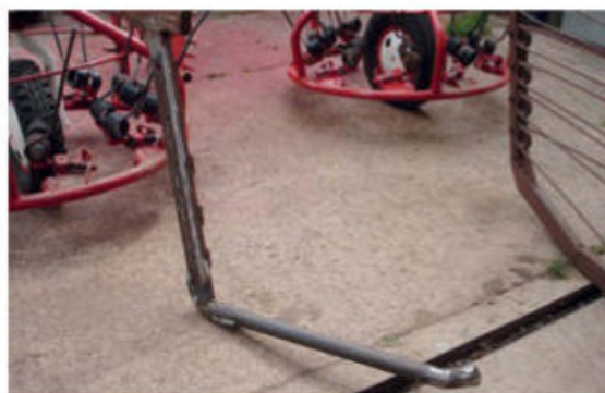
Just got the gates to sort out and then nearing the end of the repairs.
