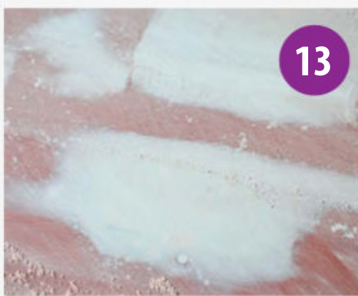
Rub down using a sanding block going through the grades.
