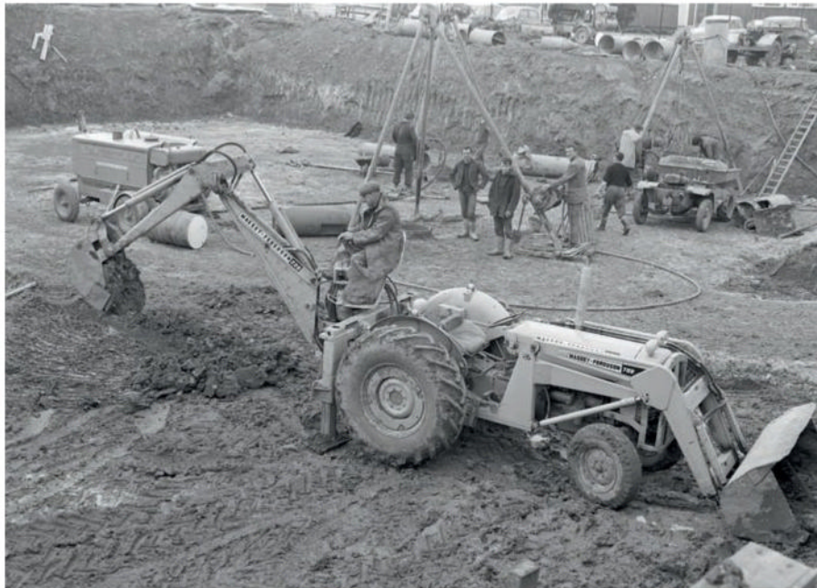
Construction on the Banner Lane tower block started in 1965, it was opened in 1964.
