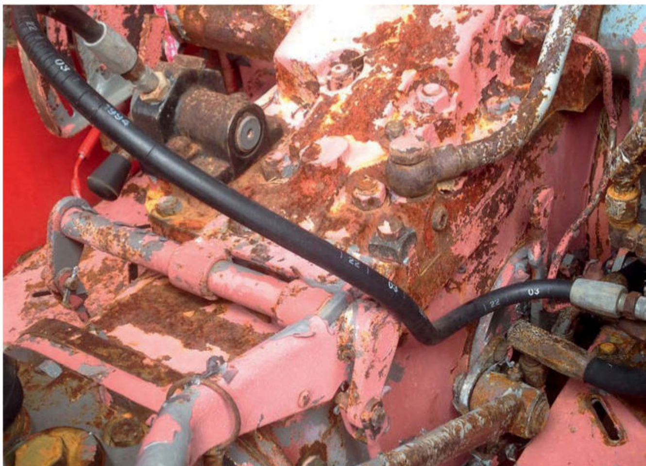
One session with the steam cleaner was sufficient to lift the grey paint and reveal this odd shade of pink primer.
