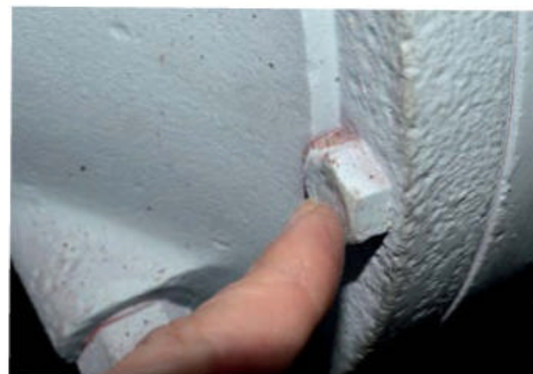
To reach the outer seals, I needed to remove the hub and this meant undoing another collection of nuts and bolts...
