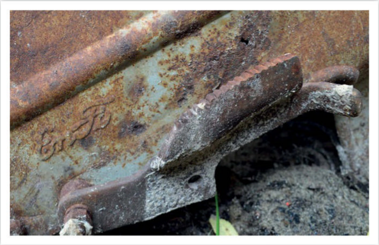
The pawl locates on this catch which, in turn, is attached to the wings. The grooves often wear away with the constant on/off movement, or the catch falls off the wing due to corrosion. New ones are available, though.
