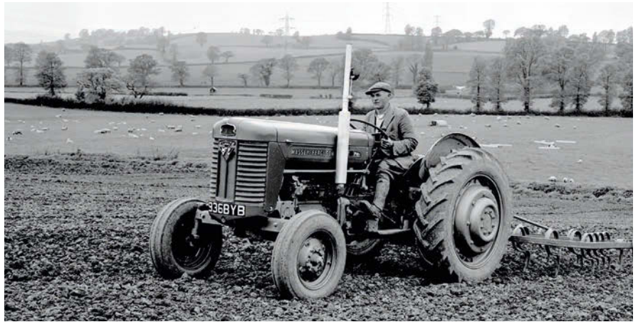
An early 65 Mk.II in action with a spring-tine cultivator. Note the shell-type fenders and tapered footplates that weren't updated until 1963. (Photo courtesy of Ted Everett)
