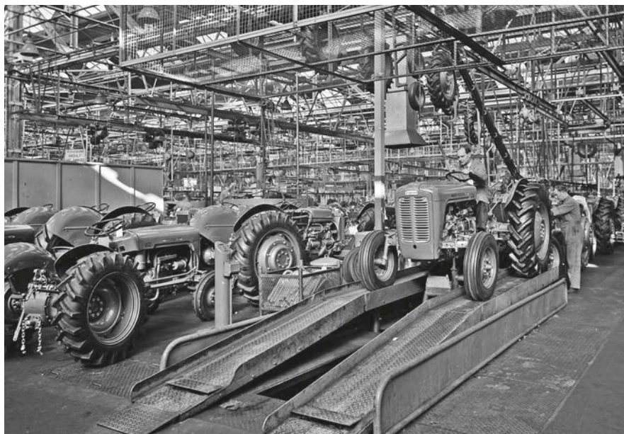
The final production line run-off point for the FE-35, circa 1957/8. Note the 35 rim on the left, that's on the wrong side of the tractor.
