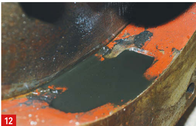
12 As I mentioned in the caption for Pic 9, more leaked oil would be visible, and it sure was! This pool of the black stuff was more than I thought there would be.
