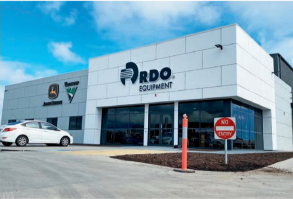
The new RDO premises in Gepps Cross
