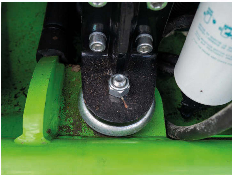
The Kubota engine mounts on the P32.6 could fail on earlier models, upgraded brackets subsequently solving the problem. Worth a periodic check to avoid the engine leaning over and causing damage, or worse still, setting on fire.
