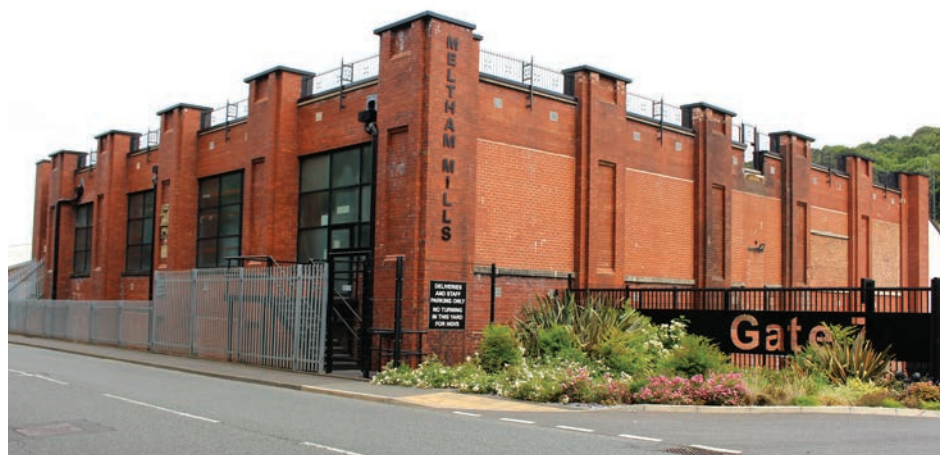
ABOVE: Another original building at Meltham that survives from DB days was originally three storeys higher and made a vital gear component for the Spitfire during WWII – thus a target for the Luftwaffe.
