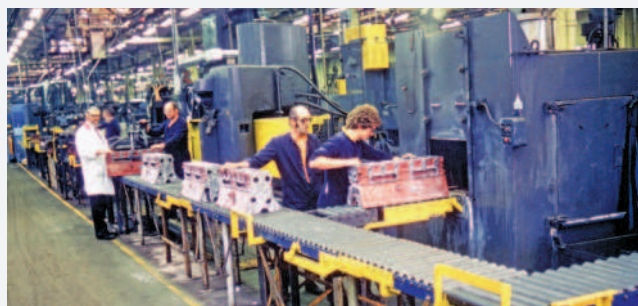
The machining line in O Block (Engine Shop) at Meltham Mills. A red collar on a white coat denoted the rank of foreman, a green collar was a chargehand, inspectors wore brown overalls and assemblers wore blue ones. Photo courtesy of Stuart Gibbard.
