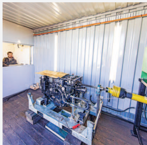
During the test cell's first run, Tom and Dan were standing ready by the stop button, but everything went according to plan.
