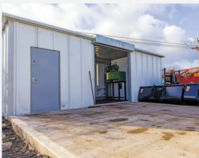
It is hard to believe the test cell building was once an old shipping container. It has been modified, insulated for noise and finished off with cladding to become a dedicated transmission test cell.
