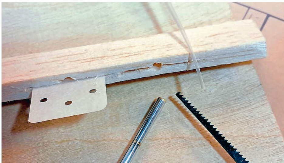
Using the fine pull-saw to cut hinge slots is easy and quick. The pilot hole is perfect for wicking-in cyano for a good hinge/wood bond.
