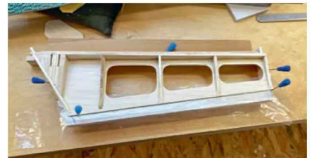
One of the elevator halves under construction. Horns are glued to the plywood ribs, seen on the inward side. Although designed to take two horns, in the end one sufficed.
