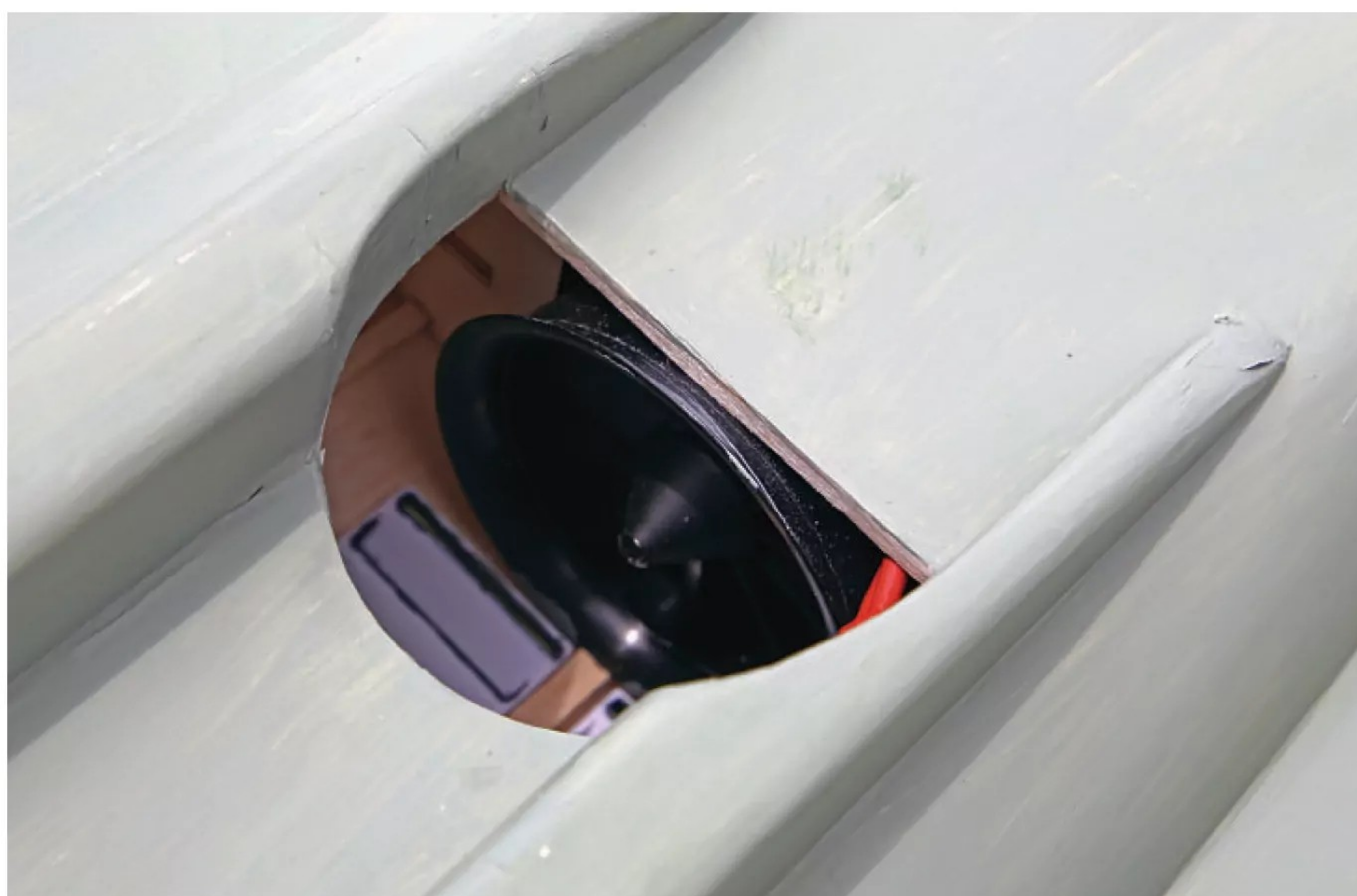
With the fan installed a portion of the removed air intake can be glued back into position behind F7.
