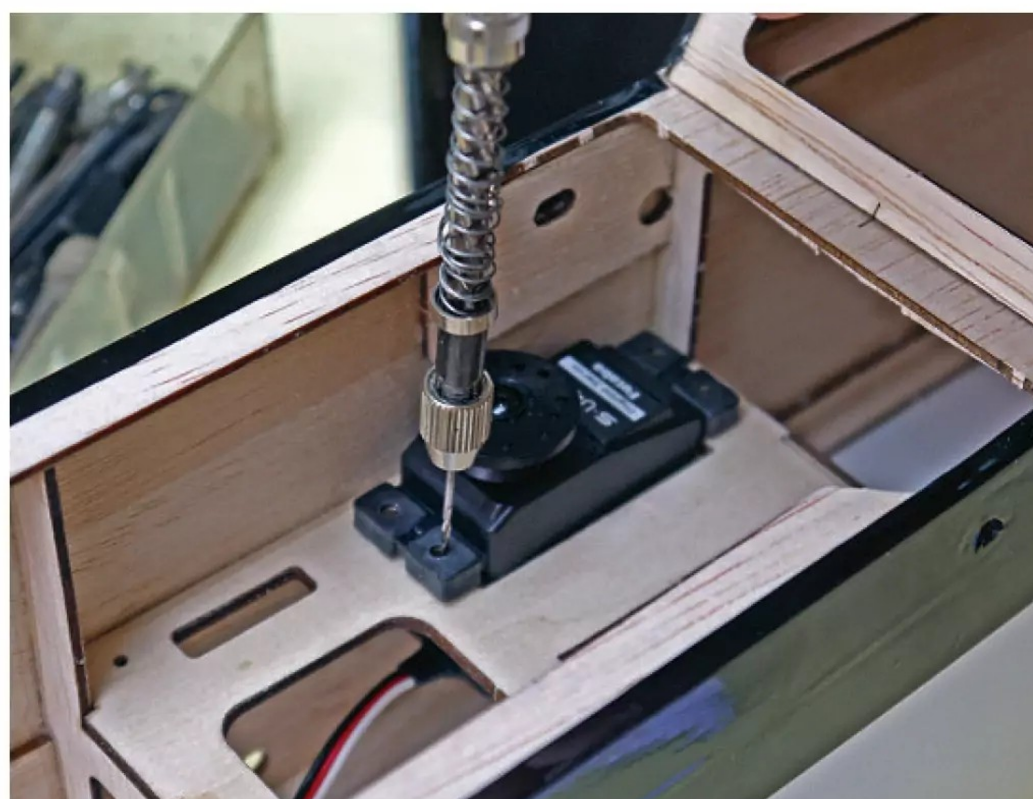
A pin drill was used to drill pilot holes for the tail servo mounting screws.
