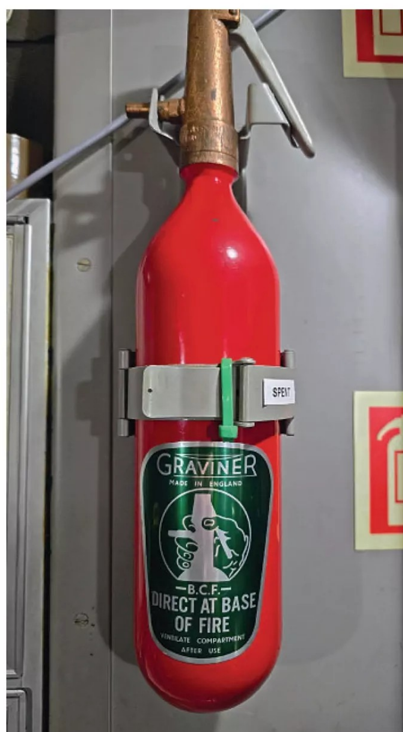
Graviner Fire Extinguisher. The museum is three short of the four that should be fitted to the Nimrod.
