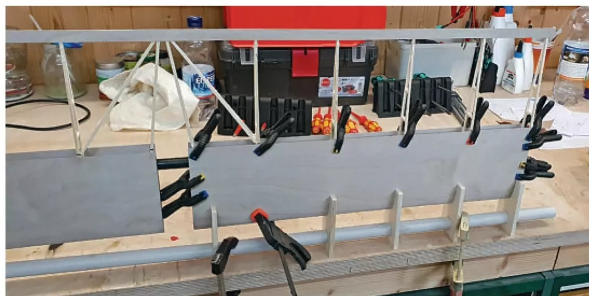
Installing the thin ply sheeting with the help of negative forms.
