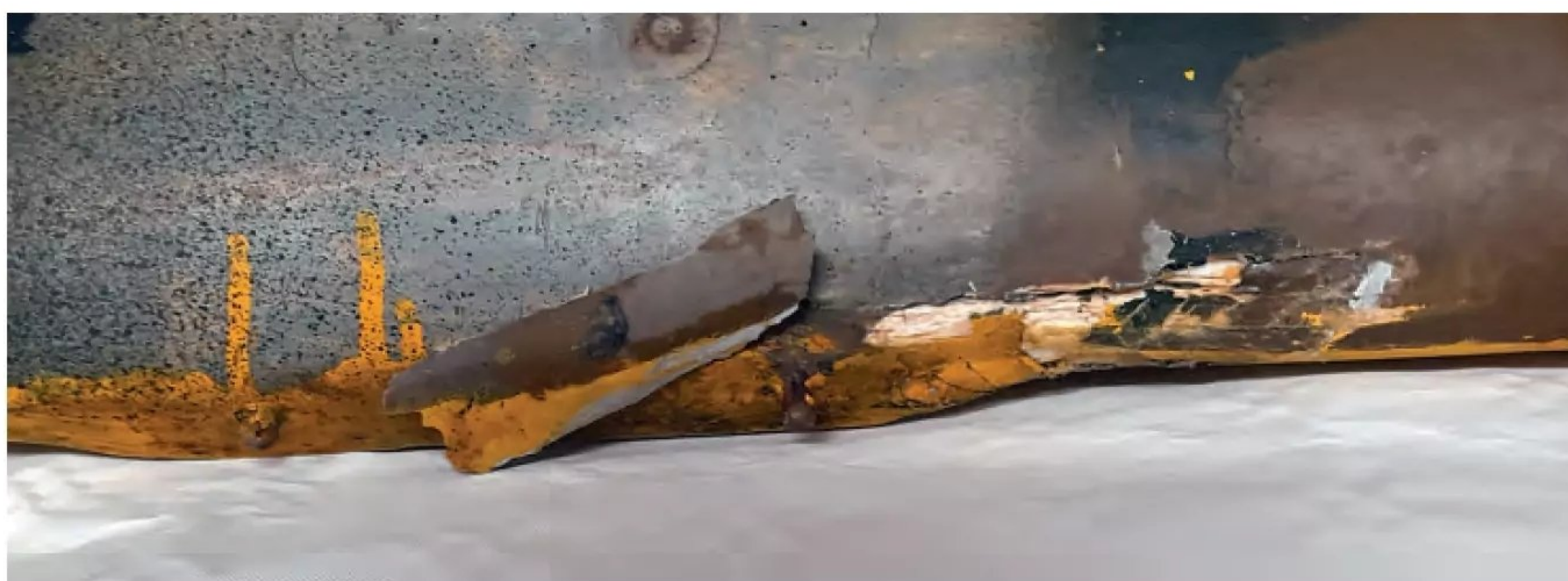
A crushed section of leading edge was cut out and new wood spliced in.
