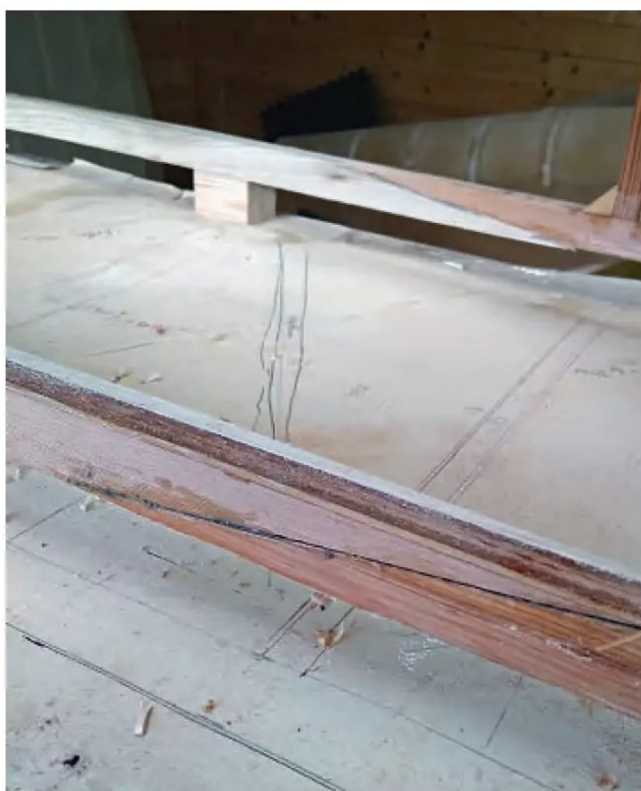
Ian carefully cut the splices in the longerons using a slope of 12 to 1, making sure the angles on the corners were at 90 degrees.
