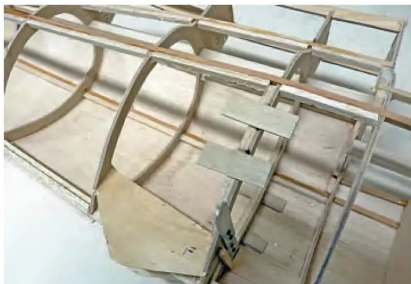
View of strut mount and wheel box. Note the ply transfer plates.
