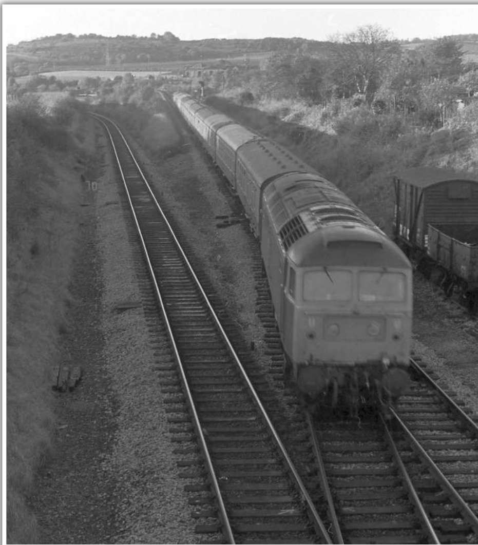
Princes Risborough, June 1982. An unidentified Class 47 coasts down the grade towards the station. The variation between the Up and Down lines can be clearly seen (the tunnel and cutting are round the curve to the left). At this time the station was reduced to one usable platform, which often resulted in passing movements on the approach.
