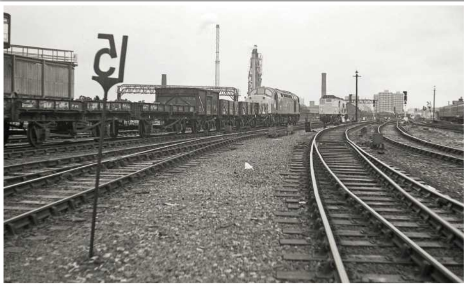
Returning from its banking duties, 25049 passes 40020 which is making an unaided ascent to Miles Platting with a Warrington Arpley to Healey Mills freight on 24th September 1975.
