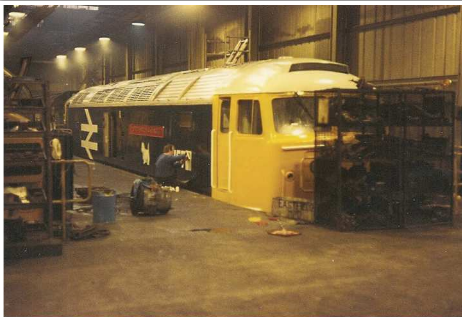
Painter Jim Kerr applies the numbers to 47578 in a smoky shed at Eastfield on January 22nd 1985. The black window surrounds and black headcode panel are yet to be applied. Note the hand painted BR logo. 47578 was named 'The Royal Society of Edinburgh' at Edinburgh Waverley four days later.
