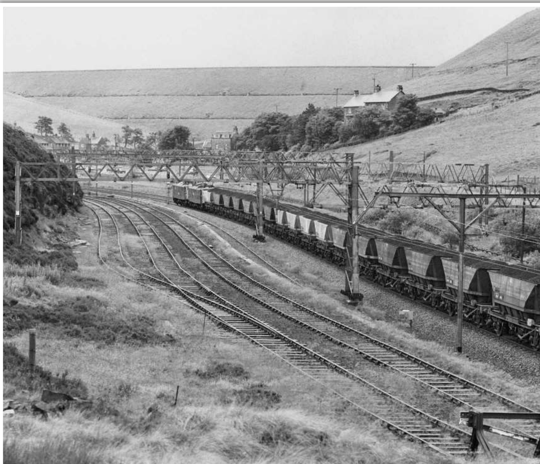
17th July 1981: Following 76051 into Woodhead Tunnel were 76012 and 76007 on another westbound MGR service from Barnsley Junction, the next duty for the pair of 76s after Worsbrough banking work in the morning. I would have assumed that they had assisted 6M21 through to Barnsley Junction, but photographic evidence on the web shows them arriving there light engine, suggesting they had dropped off the back of the train at West Silkstone Junction as normal. Prominent in the going away shot is the dam wall of Winscar Reservoir (1975) which dominates the few houses constituting Dunford Bridge.
