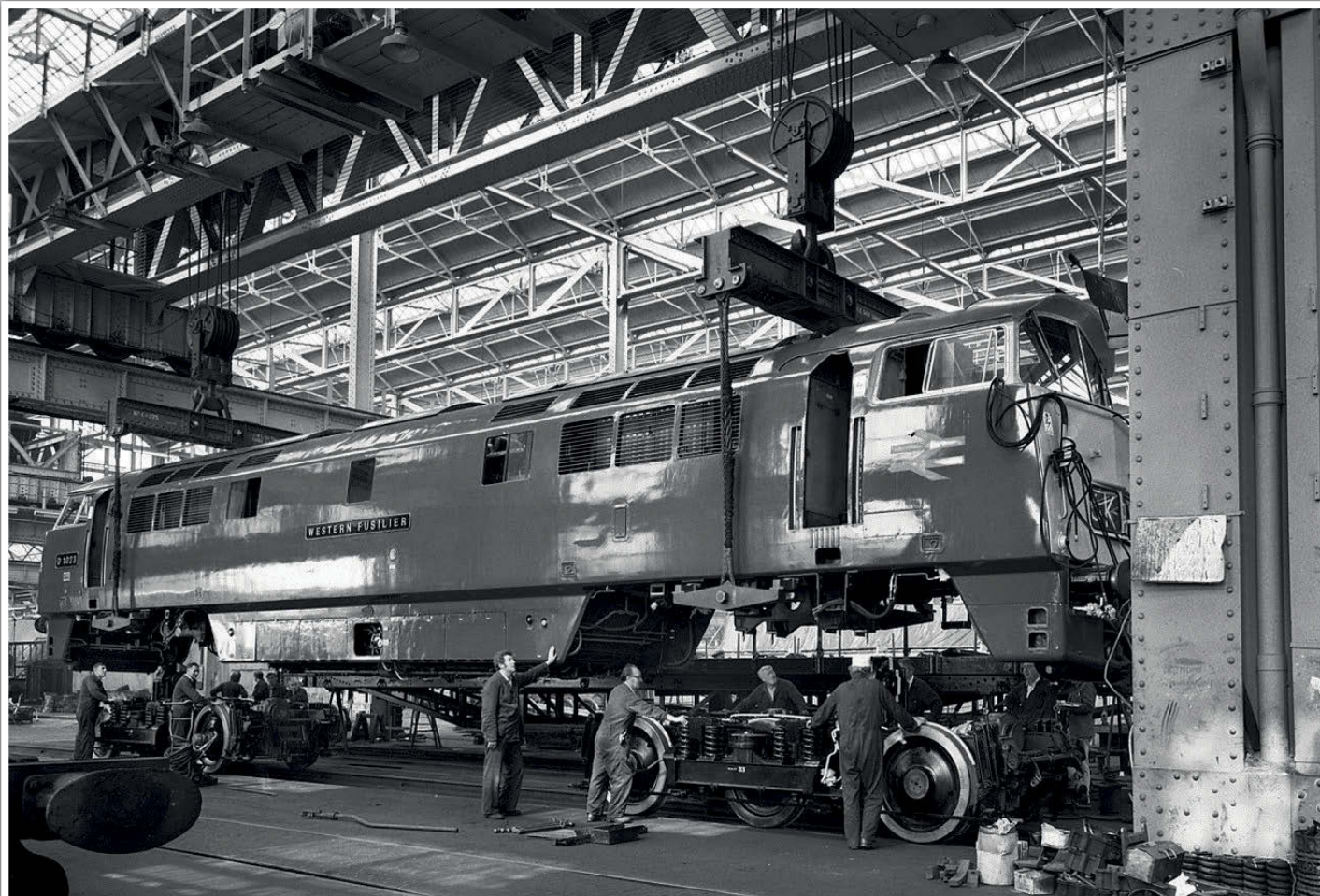
D1013 'Western Ranger' is lowered onto its bogies after overhaul at Swindon Works. COLIN MARSDEN
