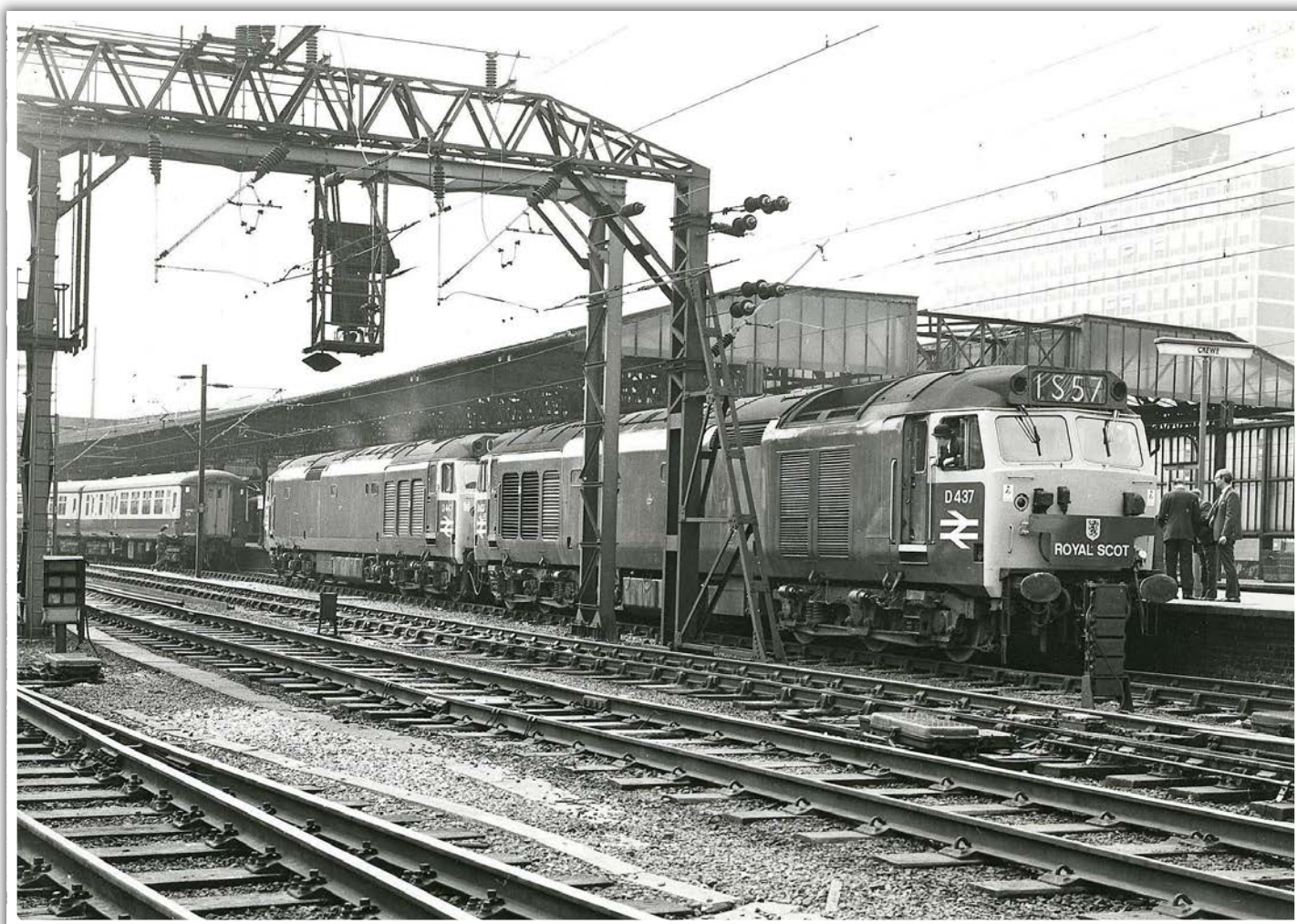
Changing traction from electric to diesel at Crewe involved the Class 50s leaving the depot and running nearly to Crewe Coal Yard to await the removal of the electric locomotive before backing onto the train. On 4th May 1970, the inaugural down 'Royal Scot' of the twin-Class 50 era, with 447 and 437 in charge, carried a headboard. The pair are seen backing onto the train at Crewe. DAVID CLOUGH COLLECTION
