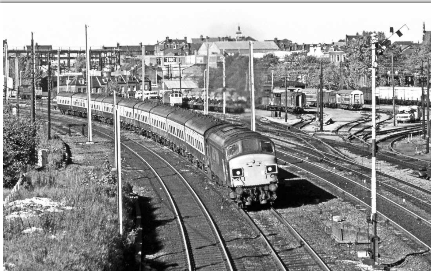
Circa 1981: Crawley Green road bridge, to the south of Luton station, afforded good photogenic views of southbound trains, but all this was about to change with the then forthcoming 'Bed-Pan' electrification (note the electrification masts). A 'split-box' Class 45 'Peak' (believed to be 45120) heads for the capital with an 'Up' express. A couple of Class 25s are also visible and Crescent Road Goods looks to contain a healthy volume of traffic, which includes Bedford truck chassis and international ferry vans, the latter including refrigerated types (far right) used for perishables such as fruits, meats and vegetables. Believed to be one of the last flows using refrigerated wagons in the UK these were for the import movement of offal to Melton Mowbray for Pedigree Petfoods, which ceased circa 1990 (a colour version of this image can be found on Kevin's 'Lost-Albion' Flickr site).
