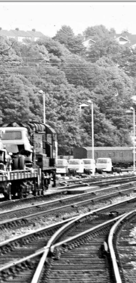
(LEFT) August 1975: A major source of rail freight traffic generated in the Luton area was provided by the automotive industry. A raft of 'auto-flats' laden with a mixture of Bedford TK trucks and Vauxhall cars are shunted by an unidentified Class 08, although the white truck is actually a Ford 'D'. Further Ford 'D' types can also be seen in the background standing in Crescent Road Goods Yard (a colour version of this image can be found on Kevin's 'Lost-Albion' Flickr site).
