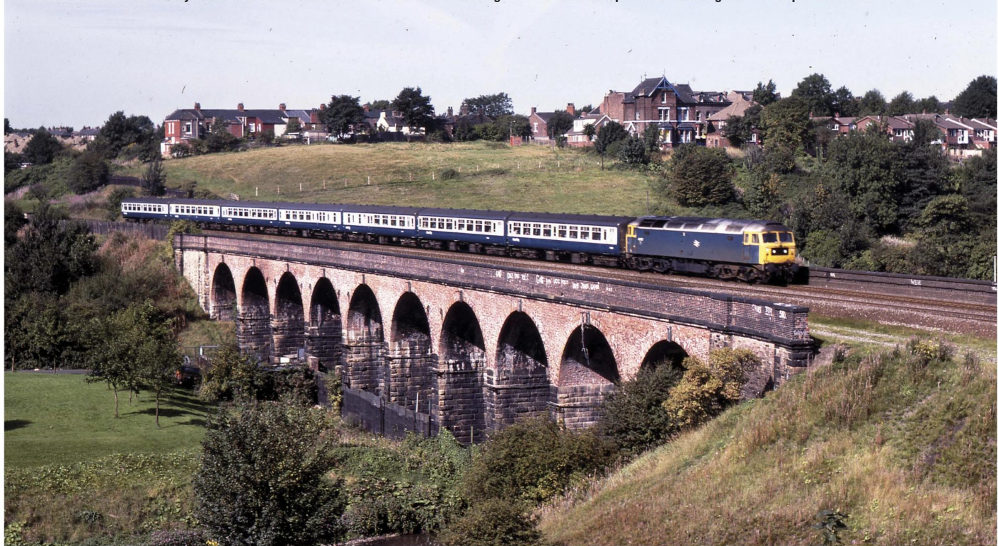
Medlock Vale viaduct near Droylesden sees Gateshead's Class 47/7 No. 47557 crossing with the 11:05 Liverpool to Scarborough on 11th September 1982.
