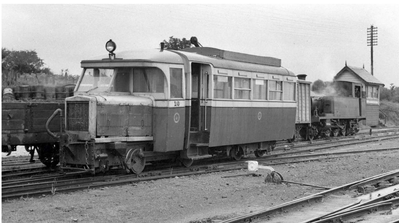
This is the vehicle that started it all! Railcar 10 of the County Donegal Railways, formerly No. 1 of the Clougher Valley Railway, took the author across the border to Stranorlar, where it is seen resting briefly in summer 1956. The power bogie at the front carries the engine, gearbox, driving cab and controls; the passenger saloon is articulated off it.
