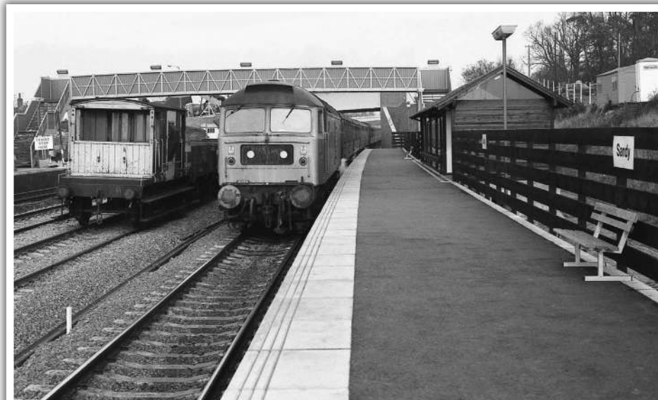
(ABOVE) 47024 passes through the new southbound platform at Sandy with an express. Maintenance wagons occupied the Up Fast at this time.
