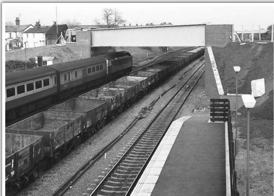
47428 passes slowly through Sandy with a down express. At this stage only part of the track re-alignment had been completed. Maintenance wagons occupied the Up Fast line. The picture was taken from the new southbound platform, which stands on the site of the former LNWR station. The new single span A603 road bridge was already in place.
