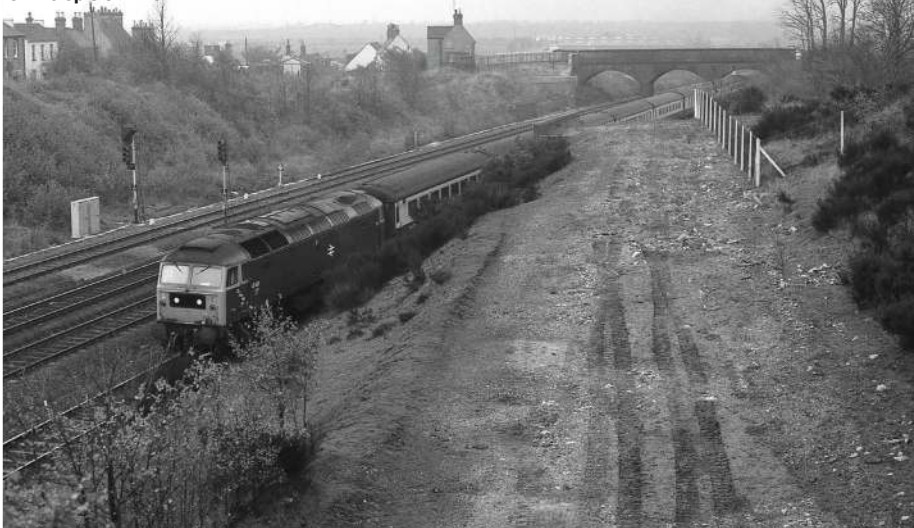
47423 passes the site of the former Bedford line flyover, with a southbound express on the Up Slow line.
