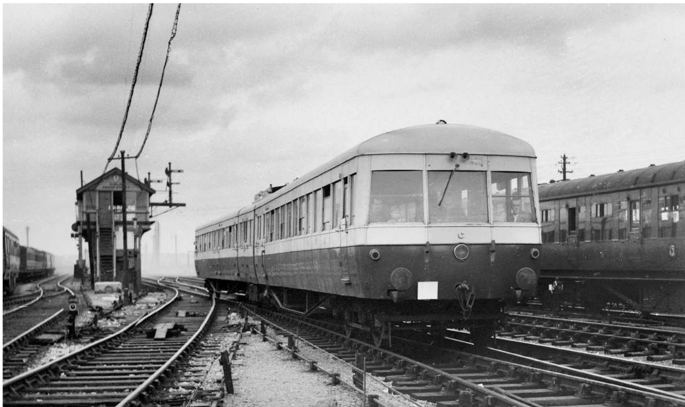
There is a prototype for everything! Arriving at Dublin Amiens Street station (now called Connolly) in July 1957 on a suburban service from Howth is Great Northern Railway railcar G, a two-car set with central power pod. The power unit rides on two axles, with the passenger cars articulated off it. This set, together with its twin railcar F, was built in 1938.
