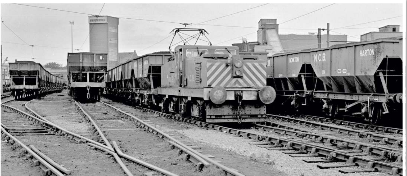
(BELOW) No. 12 buffers up to a rake of loaded coal wagons for transit to the St Hilda sidings, where the rake will be split into three eight-wagon sections for the steep drop through the tunnel to Harton. COLIN BOOCOCK
