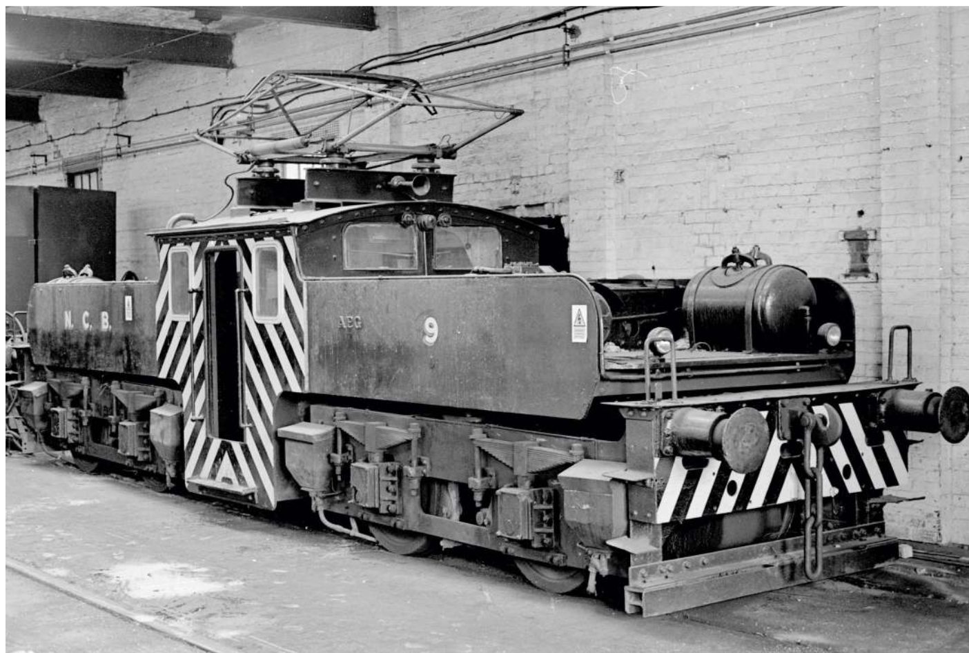
AEG, also of Germany, delivered a single Bo-Bo electric locomotive in 1913, No. 9. This served the railway for longer than the Siemens machines; it was still operational at the time of the author's visit in late 1987 and was sitting in Westoe depot. The locomotive is now stored in the open at the Tanfield Railway. COLIN BOOCOCK
