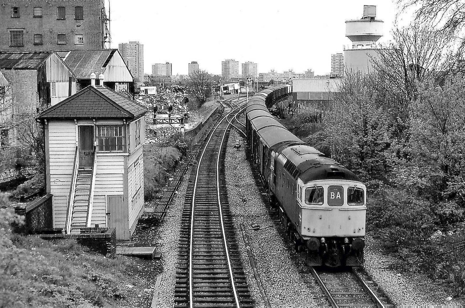
(ABOVE) Monday 7th May 1979: Having crossed the River Thames by means of Cremorne Bridge (a Grade 2 listed structure dating from 1863), 'Slim Jim' 33212 passes Chelsea & Fulham signalbox and the connection leading to Chelsea Basin Goods (closed in 1981) with a long raft of Continental vans (including refrigerated types), which have most likely originated from Dover. Indeed, the service could well be 6S73, the 11:00 Anglo-Scottish Speedlink service from Dover to Dundee, which called at the major West Coast Main Line yards at Willesden, Bescot, Warrington, Carlisle and Mossend. The traffic stop at Willesden may entail detaching vanloads of perishables (imported fruits and vegetables) for onward movement to Stratford LIFT and/or perhaps for working back over the WLL to South Lambeth Goods. STEPHEN BURDETT.
