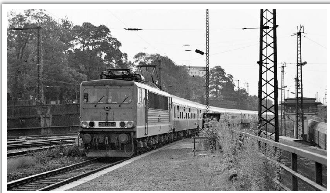
Two Deutsche Reichsbahn Bo-Bo electrics are seen stabled outside Dresden Hbf in 1992. On the right is 242 001, the first member of the earliest post-war DR freight electric locomotive of Class E42 that later became 242 under DR and were reclassified as 142 by Deutsche Bahn. The locomotive was built in 1963 and is now preserved. The 142s could also be seen on passenger work since speeds were generally not high in the East Germany. On the left is the newer standard mixed-traffic Bo-Bo 243 846, of a type that, after the reunification of Germany, spread across almost all of the country, running then as Class 143. Both are in the standard DR red livery. COLIN BOOCCOCK
