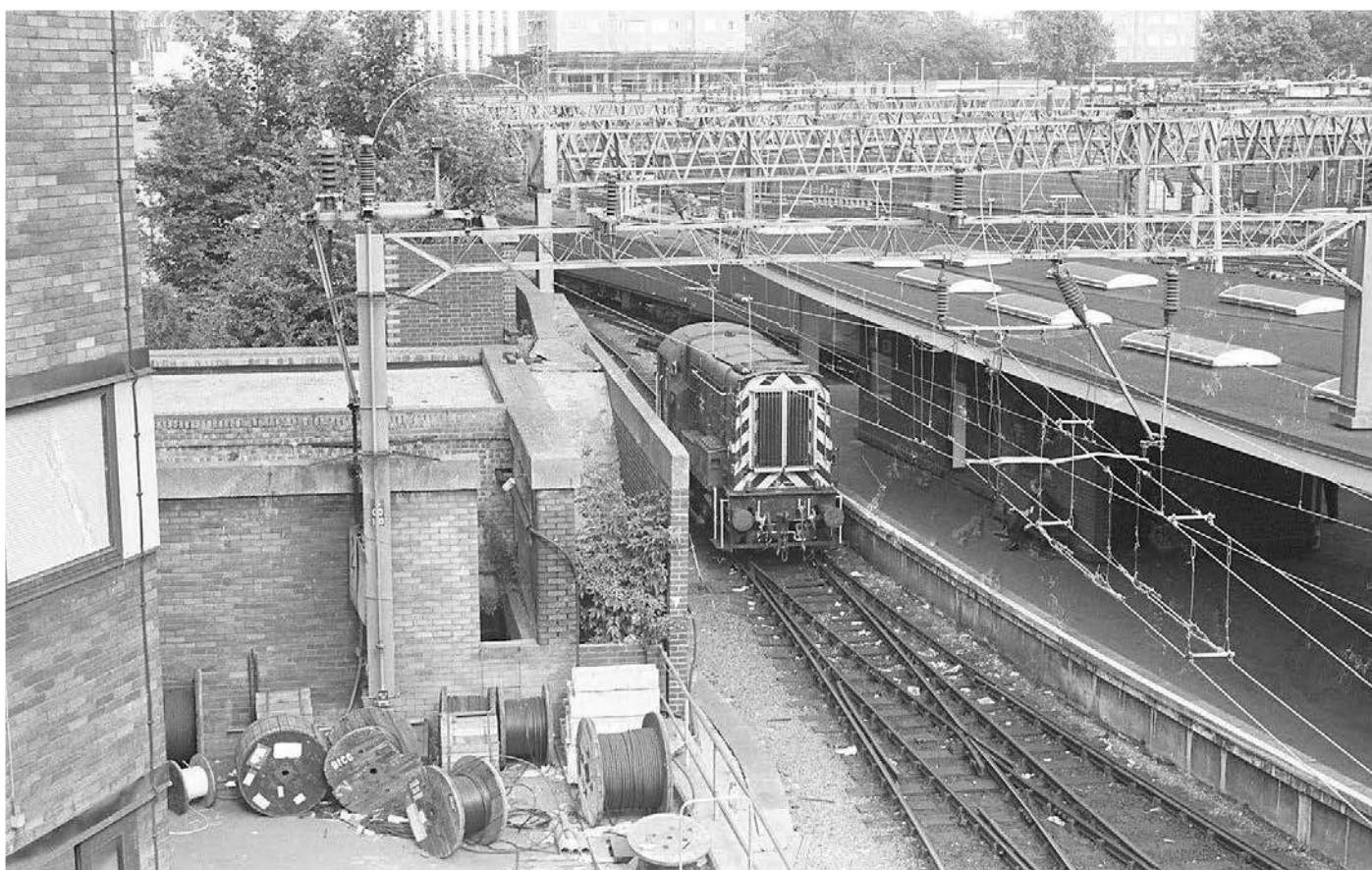
A daytime view of the parcels side of Euston with 08454 on pilot duties on 17th September 1985. The '08' is alongside the yard supervisor's office. The building also housed the engine arranger's office and a small area which I believe was referred to as 'The Ferry Cabin' for train crews. It is possibly a driver who is taking a break sitting outside on the platform. The parcels area of the station was made up of platforms 18, 19 and 20, with platform 19 having platform faces on either side. The 'unofficial' walking route to the signal box was along this platform. The three way point in front of the locomotive leads to the lines known as Short Dock 1 and 2. The windows of Euston PSB can be seen on the left. JOSEPH PORTER: IVAN STEWART COLLECTION
