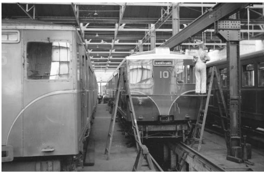
(ABOVE) Inside the upper storey of the LOR workshops at Seaforth Sands is car 10 as part of a three-car unit nearing the end of its rebuild in summer 1955. Only eighteen months later the railway would close. Even though it was profitable, the company could not afford the cost of repairs to the overhead structure and decking. COLIN BOOCCOCK
