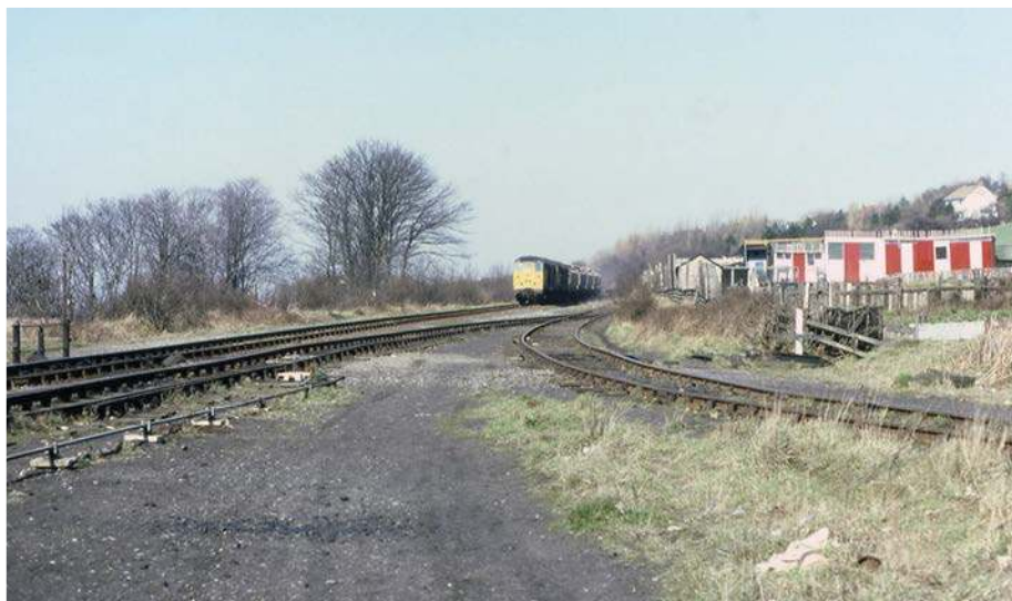
On Thursday 25th March 1982, two Thornaby Class 31s, Nos. 31178 and 31292, drift down past the entrance to the still operational Brotton coal depot. The line to the right of the running line required an Annets key to release the ground frame that controlled access. This was obtained from Longbeck signal box at Marske.
