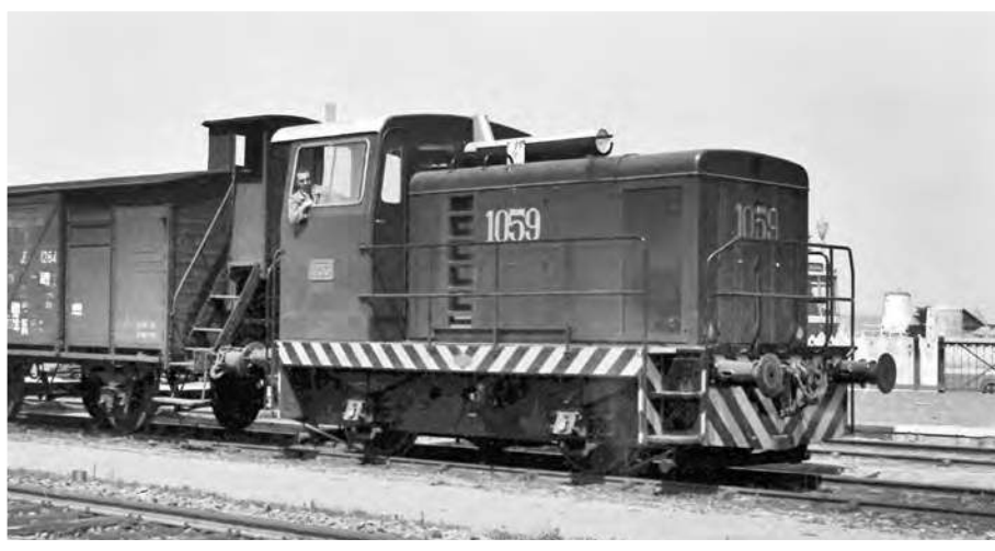
A batch of eight four-wheeled diesel electric shunters was in use, supplied from France by Gaston-Moyes. This one, No 1059, was shunting at Barreiro, south of the Tagus opposite Lisbon.
