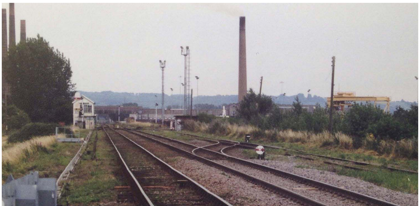
Looking west towards Bletchley, Forders sidings box is shown on the left. The lines were designated from left to right: the Up Bedford, the Down Bedford and the Forders Goods Loop. The facing points shown on the right took you into the loop once you had drawn forward past signal 36, the single disc type shunting signal. Clearance for this move was confirmed by the shunter using a two way walkie talkie.. The propelling movement then brought you to the signal number 33 with its four vertical shunt signals which can be seen alongside the shunters' cabin in the centre of the photo. With the 3rd from top disc cleared, the route led to one of the gantry roads. Two of the kilns at the brickworks are still in use. GRAHAM BAKER
