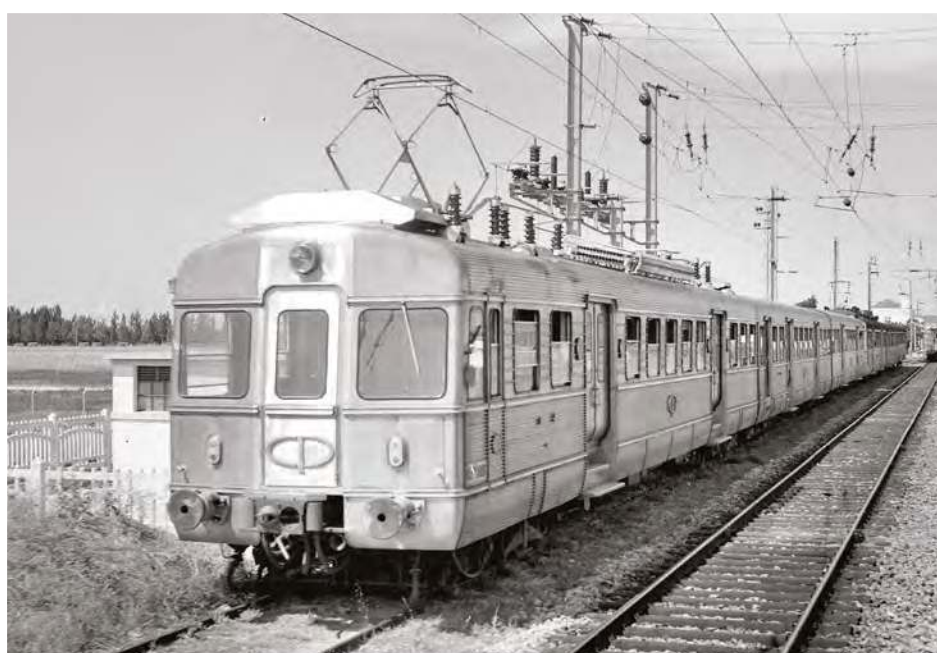
(LEFT) Two of the first batch of stainless steel EMUs that Sorefame built for CP stand outside Lisbon Apolonia station. These vehicles used a construction method patented by Budd of the USA.
