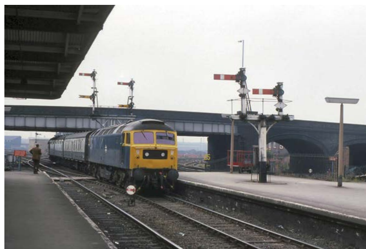
47151 runs into Masborough with a Cross Country service to York. The junction signal on the platform is another former Midland Railway timber post signal, although it has lost its pointed Midland metal finials which have been replaced with wooden caps. The crossover which this signal protects is visible in the foreground.
