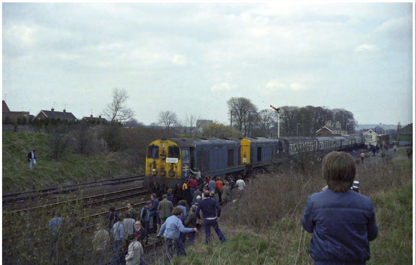
In another scene to give 21st century health and safety managers a fit, we see enthusiasts swarming all over the track and climbing into the cab of 20052 during the photo stop at Market Rasen.
