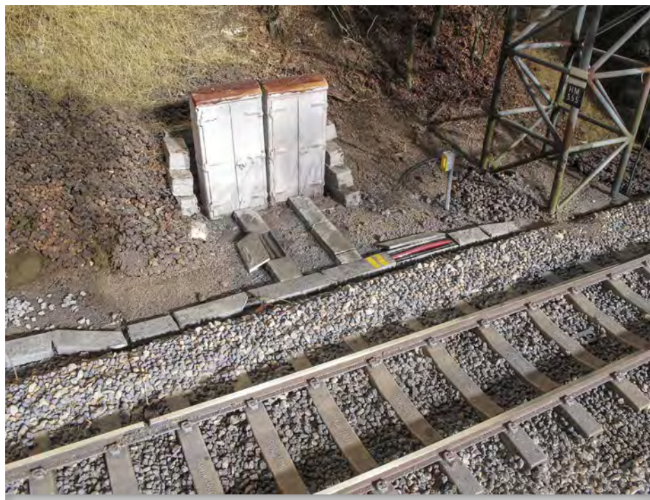
Detail shot showing the BR gantry next to Woodend Bridge. Eagle eyed readers might spot the infra red device between the sleepers in the right of the pic. This detects the passing of a train and automatically changes the aspect to red. After 30 seconds the aspect starts the sequence of going through single yellow, double yellow then green until a train passes once again. ANDY YORK
