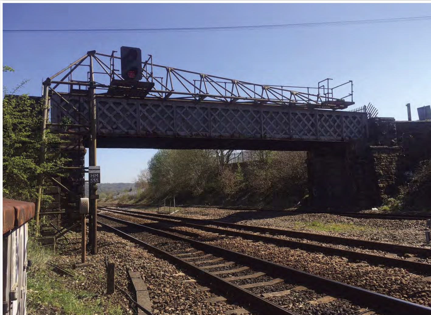
Detail shot showing the BR gantry next to Woodend Bridge. Eagle eyed readers might spot the infra red device between the sleepers in the right of the pic. This detects the passing of a train and automatically changes the aspect to red. After 30 seconds the aspect starts the sequence of going through single yellow, double yellow then green until a train passes once again. ANDY YORK
