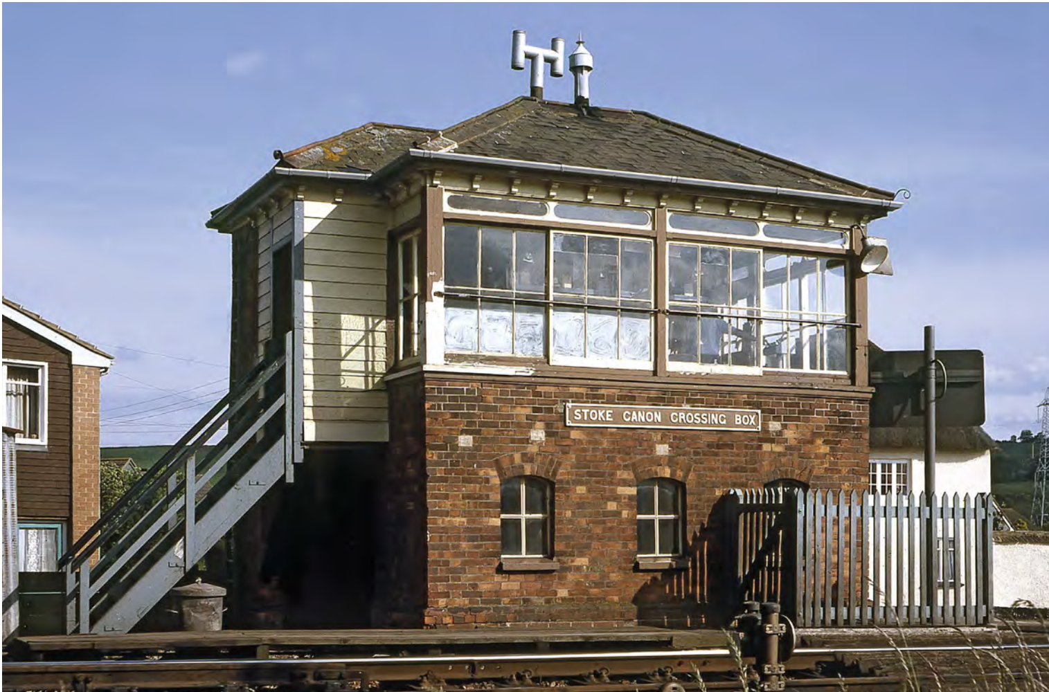
Stoke Canon Crossing signal box was a small affair built very early in 1876 by the Bristol and Exeter Railway to a design by Saxby and Farmer. It was unusual in having a row of toplight windows. It is seen here still bearing its GWR cast nameplate. Note the ground signal in the foreground guarding the crossovers. 1st August 1979
