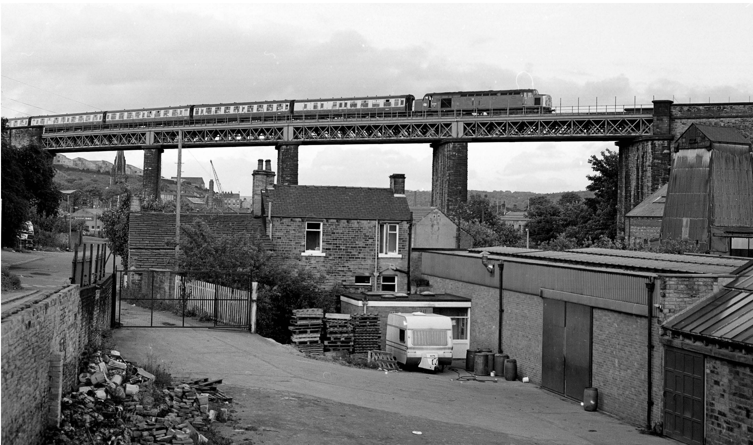
BELOW: The Penistone line diverges from the main Leeds to Manchester route at Springwood Junction at the end of Huddersfield tunnel and, almost immediately, crosses the Colne Valley on Paddock Viaduct. Class 40 No. 40001 is seen crossing the viaduct on a returning Blackpool to Penistone special on June 26th 1983. The viaduct consists of 15 stone arches divided into two sets of 6 and 9 arches separated by four lattice girder sections.
