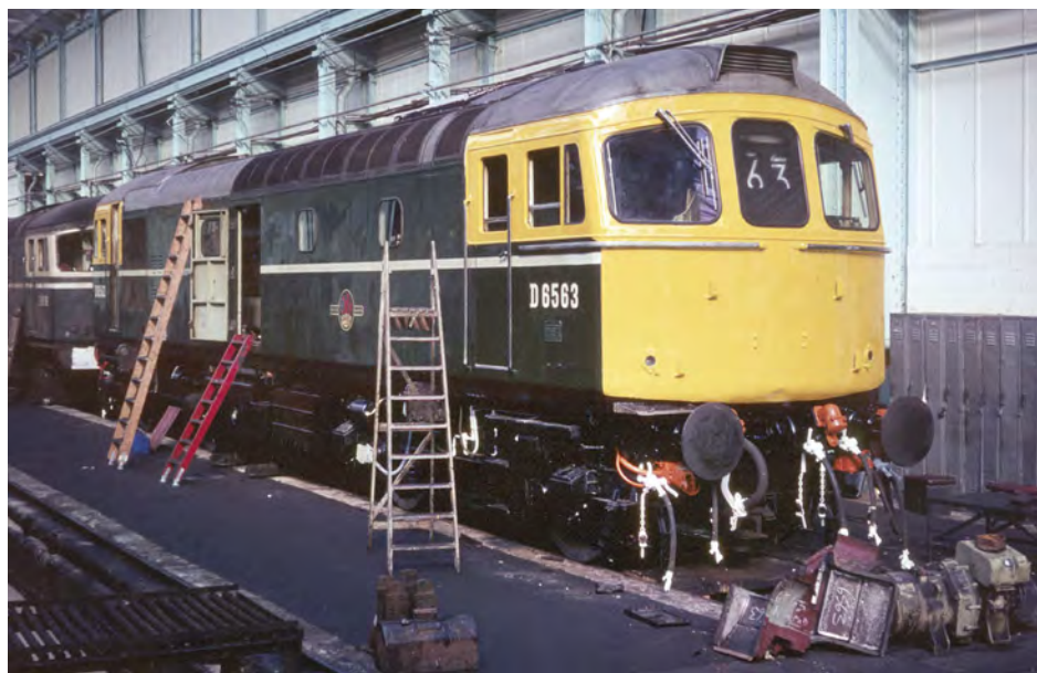
Type 3 Bo-Bo No D6563 sits in Eastleigh Works erecting shop under overhaul in 1966. On this locomotive, the progress chart based on the network analysis resource schedule is taped on the bodyside but just hidden by the long wooden ladder that reaches to the cantrail for access to the roof.
