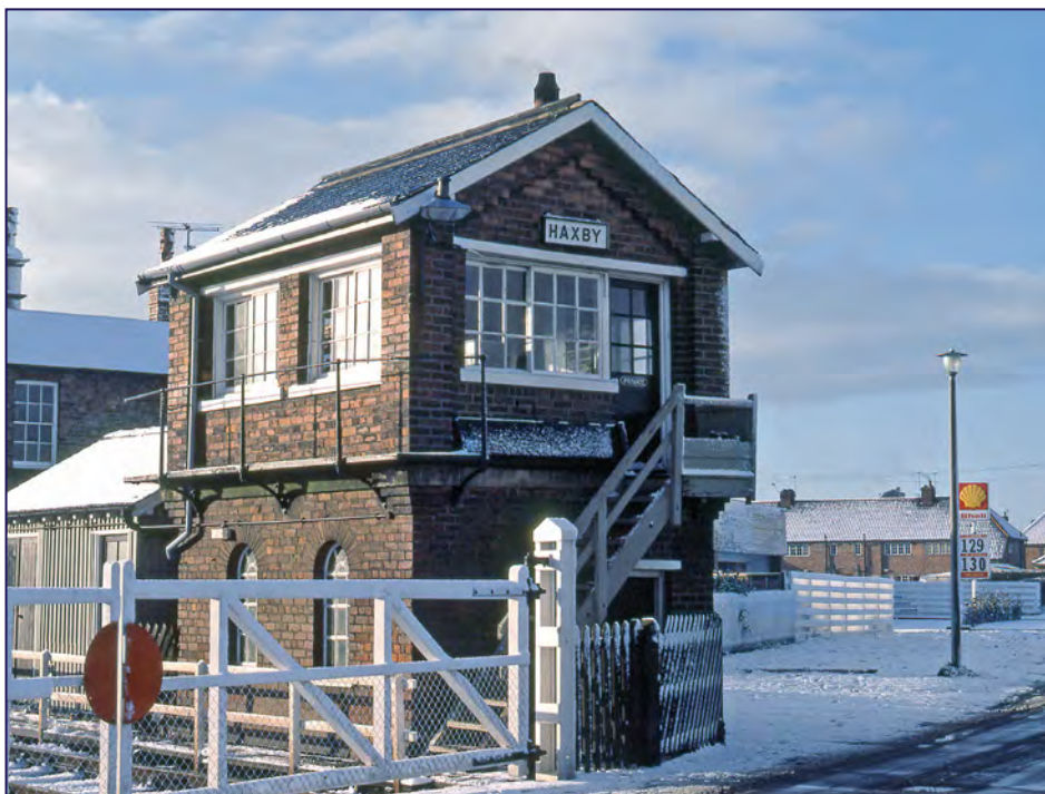
Constructed about 1878, the former NER Haxby signal box is seen in the early morning sun. It still had its manual gates at this time and a number of semaphores.
