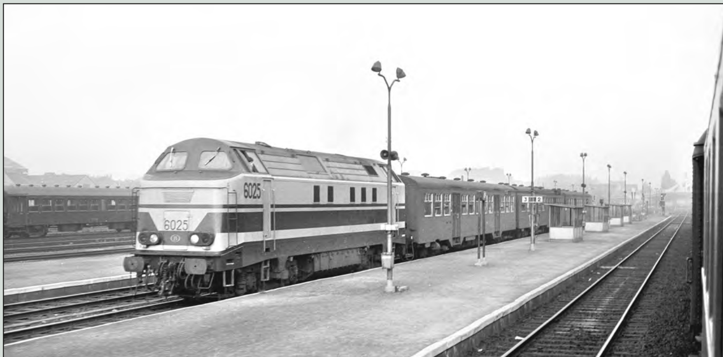
The Cockerill equivalent of the BN Class 212/62 was this type of Bo-Bo, originally Class 210 which later became Class 60. No. 6025 was photographed with a short local train at Ath, between Lille and Brussels, in 1980. This had a Baldwin diesel engine of 1,425bhp. A large number were built, 106 in total, but they were withdrawn earlier than the more reliable BN/General Motors Bo-Bos.
