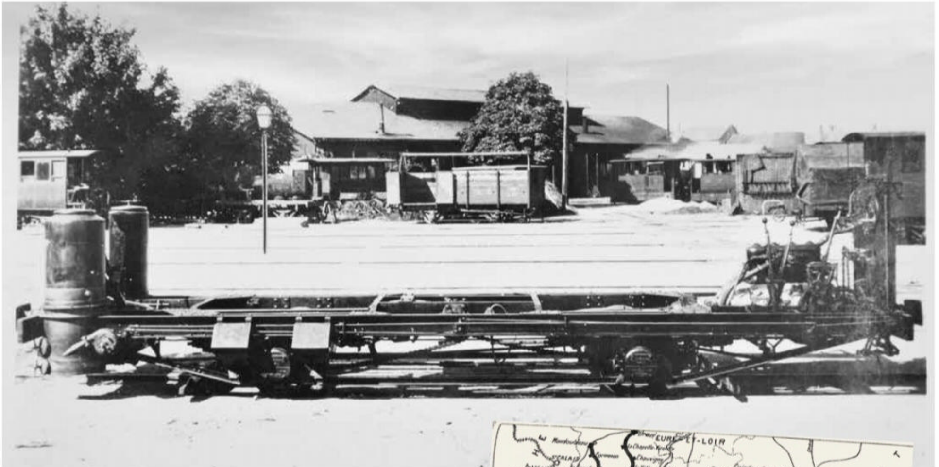
Chassis of the Panhard unit in Blois (Loir & Cher).
