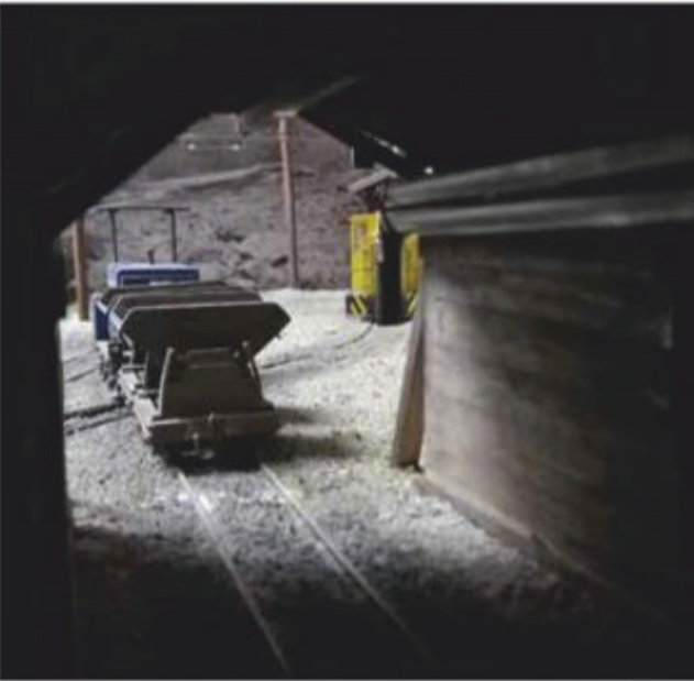
Despite being 6730m long, the tunnel has a very cramped loading gauge, its opening covers a surface of just 8.5 m²!
